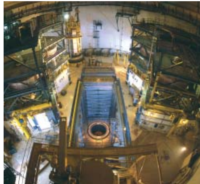
Cattenom, France (4 X 1,300 MWe): inside a reactor building.
