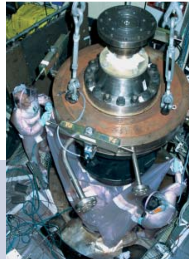
Chooz B1, France (N4, 1,500 MWe): removal of the hydraulic section of a reactor coolant pump for maintenance.
