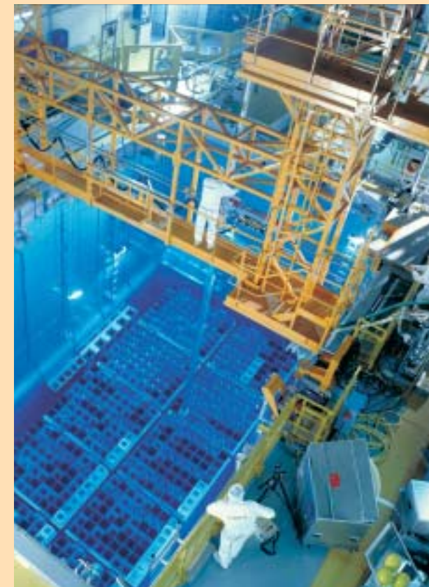
Chooz B1, France (N4, 1,500 MWe) fuel building.
