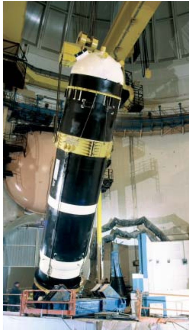
Pressurizer erection in a reactor building.
