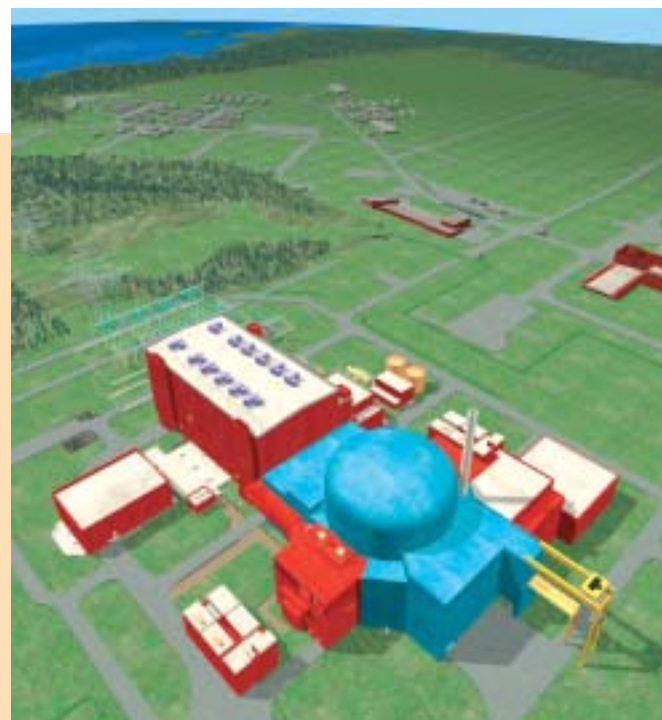
The outer shell (in blue in the image) protects the Reactor Building, the Spent Fuel Building and two of the four Safeguard Buildings including the control room.
